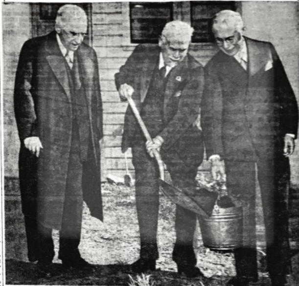
MARSHAL HALE, DR. JAMES WARD, DR. HOWARD ENGLE Dean of Old Hahnemann Hospital Turns First Spade of Earth for New Structure
